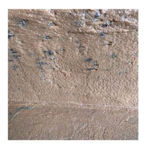
The above pictures show the applied Dampney Protexior 793 mortar. The picture on the left shows the top of the footer that is horizontal and the picture on the right shows the vertical surfaced of the footer. The picture on the right also shows the floor to footer gap; that was filled in with the Dampney Protexior 793 epoxy mortar.
