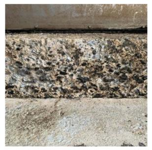
The above pictures show the concrete was prepared to an ASTM D4259 (Standard Practice for Abrading Concrete) with a surface roughness in accordance to ICRI CSP 6-8. The footing and approximately 10"-12" (254mm – 305mm) out onto the floor were prepared for the coating repair.
