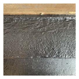
The above pictures show the finish coat of Dampney Protexior 794 applied to the concrete footing and floor area of the kiln at a dry film thickness of 4.0 - 6.0 mils (100 - 150 microns). This finish coat was chosen due to its ability to resist a wide range of acids, oils and chemical exposures and its excellent resistance to wet/dry thermal cycling when the kiln is in operation.
