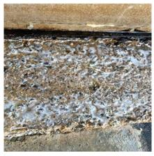
The above pictures show the concrete footing being washed with an alkaline cleaner and an all-purpose cleaner to remove any dirt residue. The alkaline cleaner was used to neutralize the acidic surface from being exposed to the tannic acid; to a neutral PH of 7. The gap at the floor to footer transition was previously caulked. The caulk was removed due to a loss of adhesion to the concrete.
